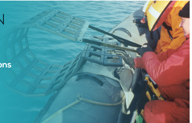
'D' Ring Patches glued with Bostik 2402 for HYPALON
